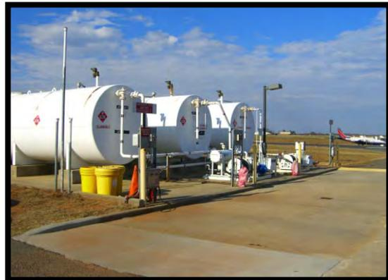
The piping, pumps, filters, and other appurtenances for the Jet-A and AVGAS tanks are located on the east end of the tank as shown in the picture. The dispenser system includes backflow lines for each tank and an automatic shutoff system to prevent accidental
