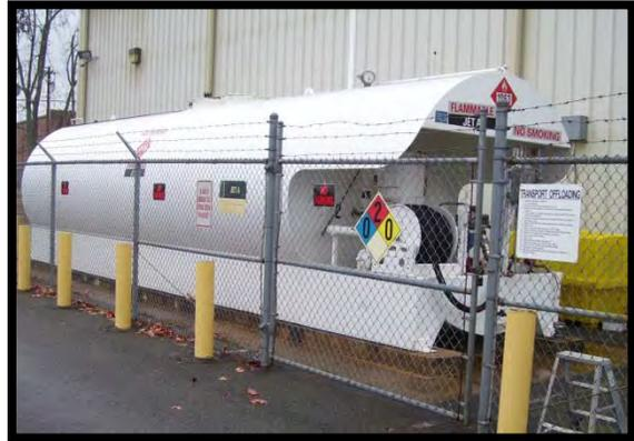
The tank is on raised skids and bolted securely to a reinforced concrete pad. The tank is painted and in good condition. The tank is double-walled with self-containment.
